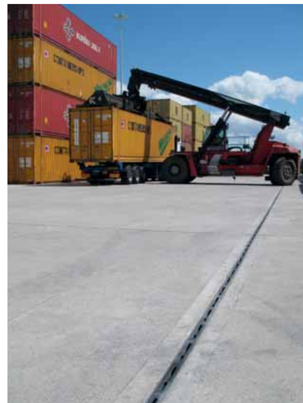
Teesport Container Terminal, Middlesbrough, UK
